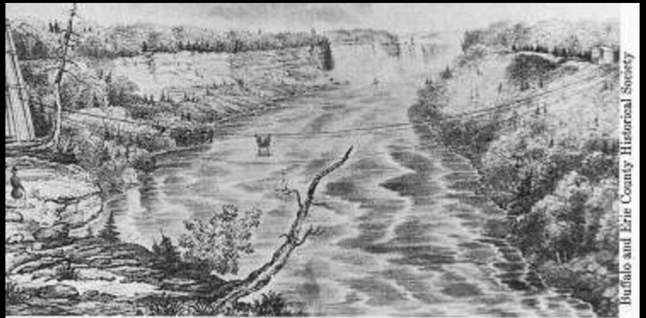
Ellett's basket, riding on cables strung between towers, 1848.
